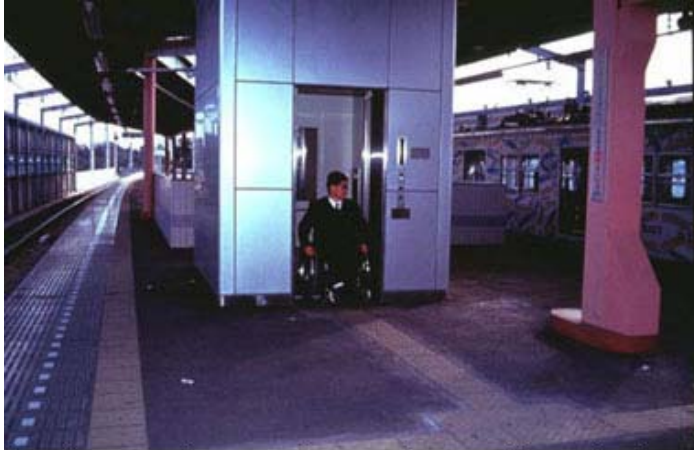
An elevator in a train station enables wheel-chair users to reach the platform on their own.
